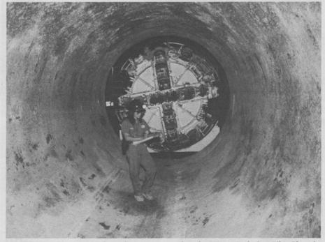
A WORKER inspects a 10-foot-diameter tunnel at the Waste Isolation Pilot Plant in southeastern New Mexico. In the background is a special tunnel-boring machine used temporarily at the site in the 1980s for brine-seepage and rock mechanics tests. (Photo courtesy of Corporate History Archives)
